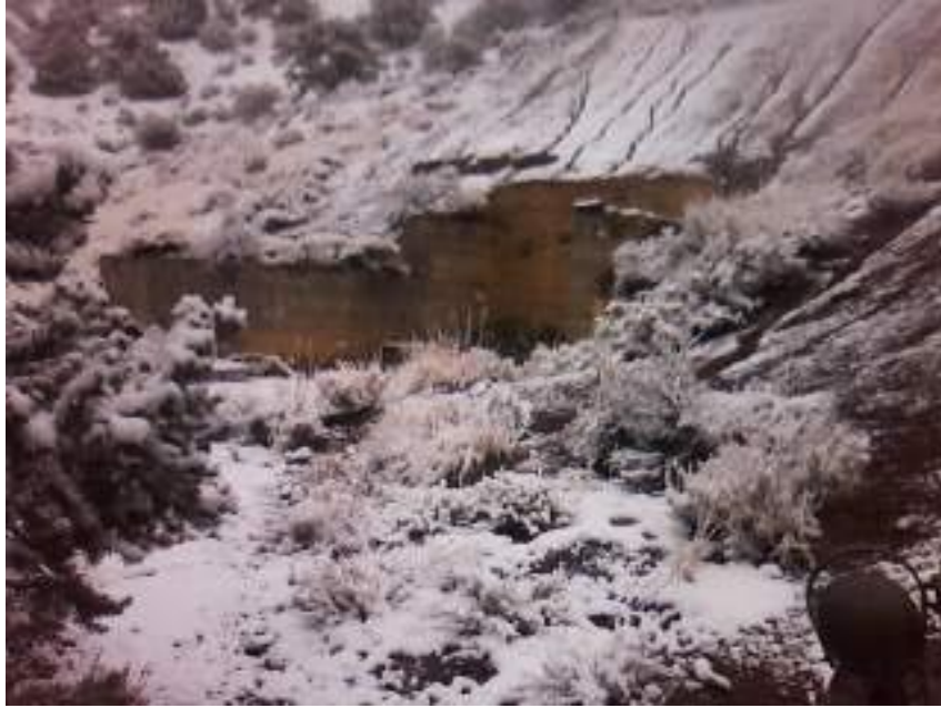
Mill foundations, Indian Queen Mine. Photo by Gregg Wilkerson, 2014
