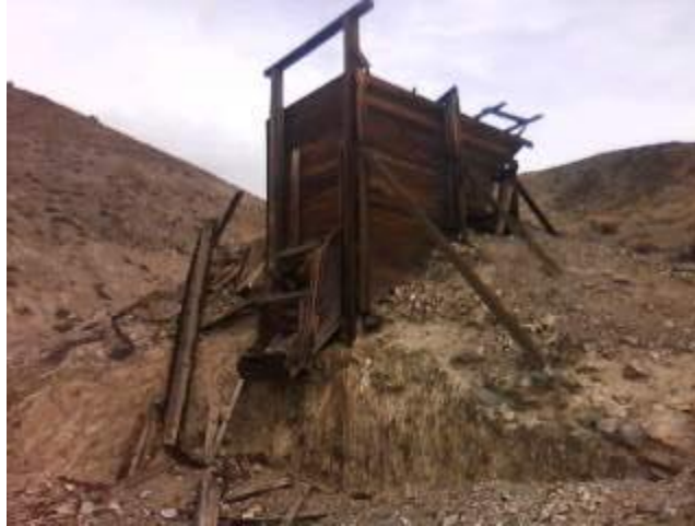
Southern Belle ore loading structure. Photo by Gregg Wilkerson, 2014
