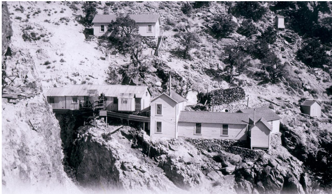
Upper mine camp of the Champion Mine, ca. 1930. All but the upper building were destroyed by fire in January 1987 (Eastern California Museum).
