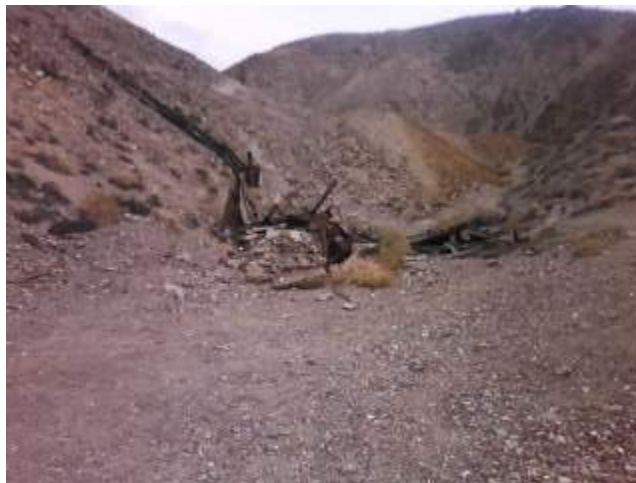
Southern Bell Mine mill site and dumps. Ore shoot delivered ore from a railroad track that connected to northern parts of the mine complex. Photo by Gregg Wilkerson, 2014.
