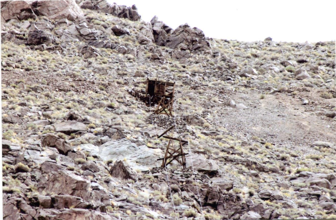
Sacramento Mine upper tramway terminal. Photo by D.D. Trent. May, 2014.
