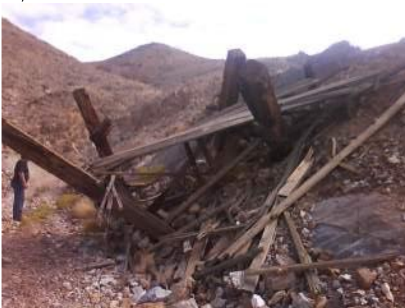
Ruins of ore lading structure, Poleta mine. Photo by Gregg Wilkerson, 2014
